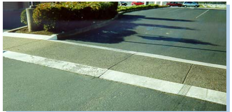
Painted, raised concrete crosswalk
