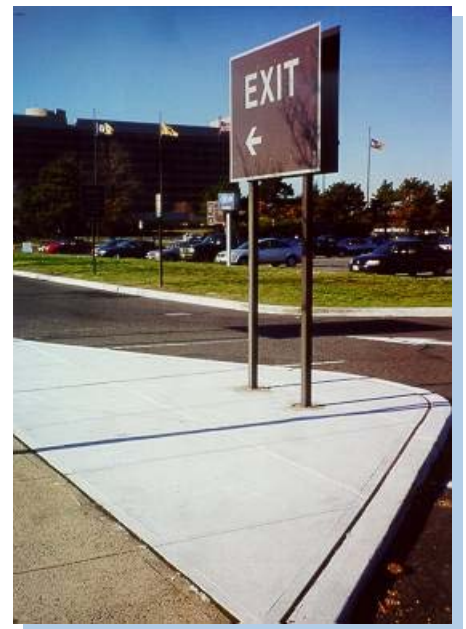
White concrete channelizer
