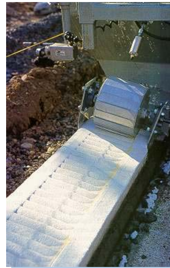
Innovative installation of reflective curbing
