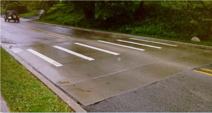
Gray concrete speed table
