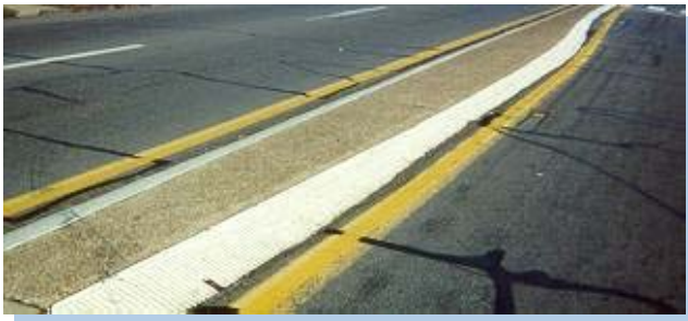
Reflective white concrete curbing, over 40 years old.
