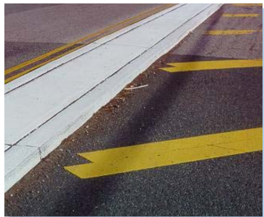
White concrete channelizer
