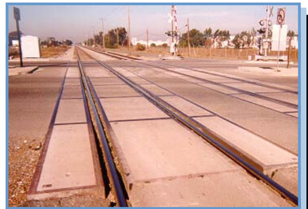
Dry precast, gray concrete. Morgan Hill, California
