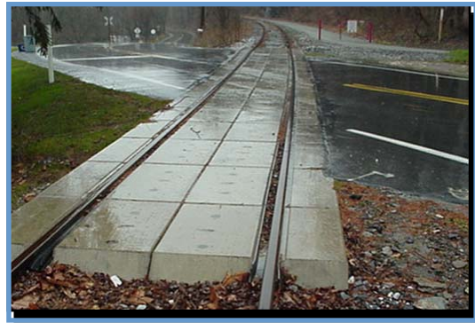
Wet precast, gray concrete. York, Pennsylvania
