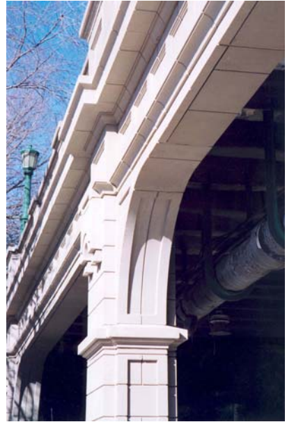
Sheridan Street Bridge, Evanston, IL
