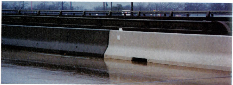
Fig. 6: Color contrast between white and gray concrete barriers increases when the concrete is wet (bottom), as this installation on I-35 in Texas shows (Photo courtesy of Lehigh Portland Cement Co.)
