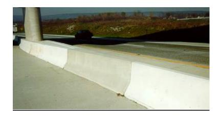
Solid fact. Bright white is the best color for maximum light reflectivity anywhere, especially where traffic safety is important. Impervious concrete median barriers made with bright white cement reflect light better – day and night – than any other kind of median barrier. **Common sense alone suggests this, and tests prove it.**
