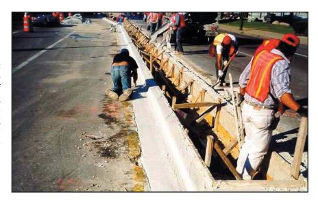
Figure 12. Standard placing and finishing techniques are used for white cement concrete, though attention to clean tools and other equipment should be exercised. (70168)
