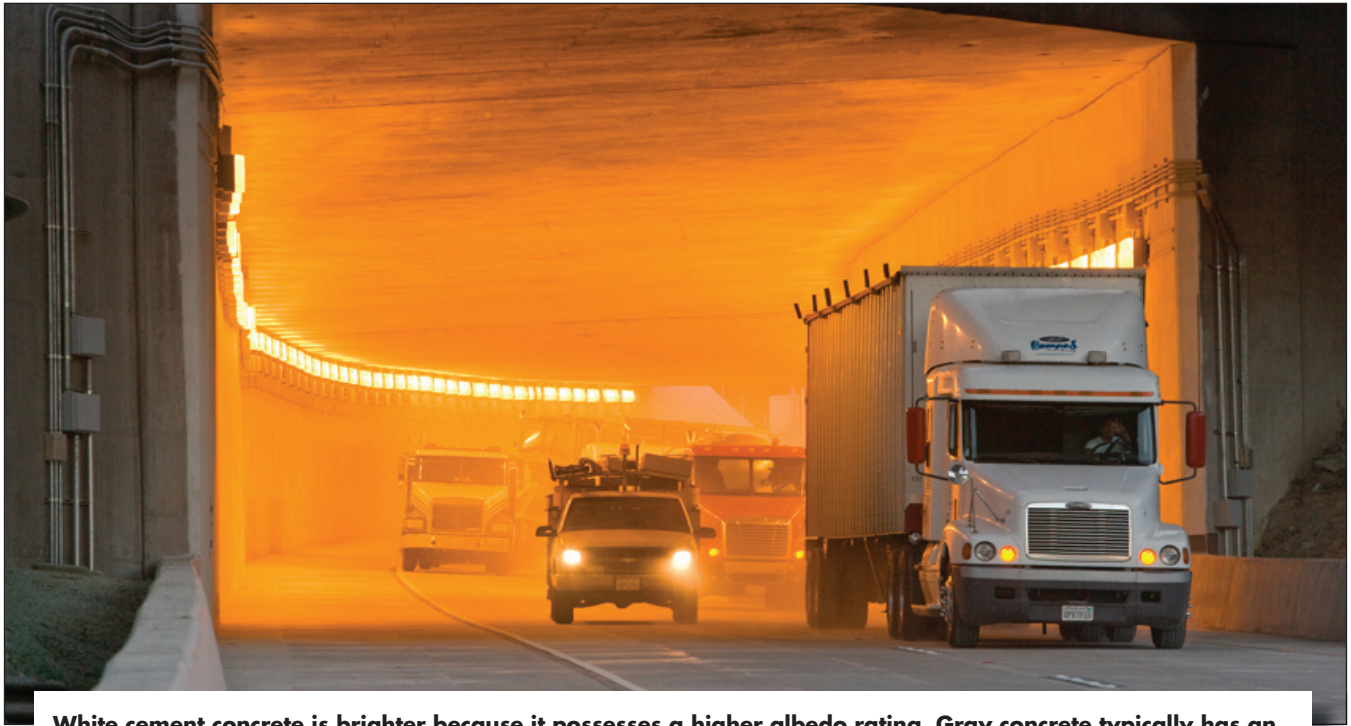
White cement concrete is brighter because it possesses a higher albedo rating. Gray concrete typically has an albedo rating of 0.3 to 0.4. White cement concrete has a rating of 0.7.
