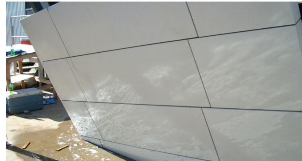
Fabrication – Finish Mock Up
