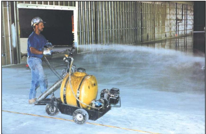
*Figure 9. A dissipating curing membrane is the preferred method of curing these white concrete floors. The membrane must be mechanically removed by scrubbing with detergent after curing is completed. (70176)*
