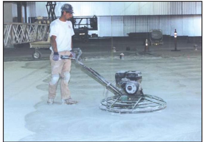
**Figure 7. A walk-behind trowel increases the speed of finishing, and changing the metal blades for different passes ensures the floor surface will look its best. (70174)**
