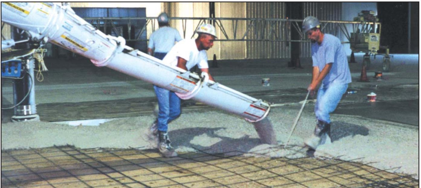
*Figure 2. With the right concrete mix, an experienced crew can cover lots of ground quickly. The placing and finishing team relies heavily on the batch plant to provide them consistent concrete from one batch to the next. (70169)*
