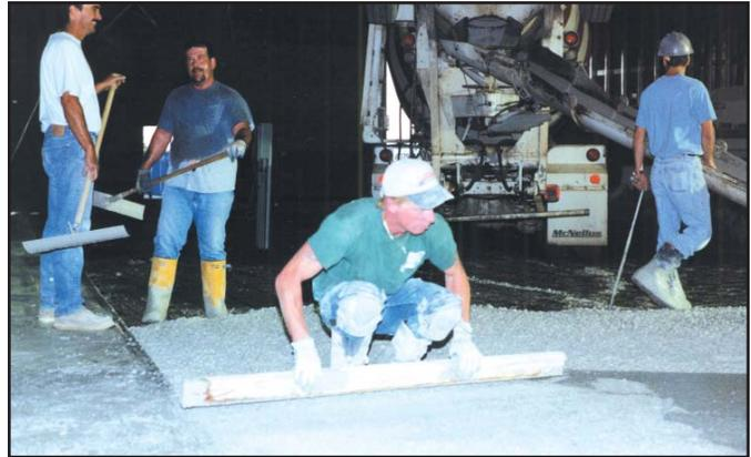
**Figures 3 and 4. For strikeoff and leveling, the finishing crew uses both advanced and simple tools, like laser screeds and wooden hand screeds, to complete their work quickly but with great accuracy. (70170, 70171)**
