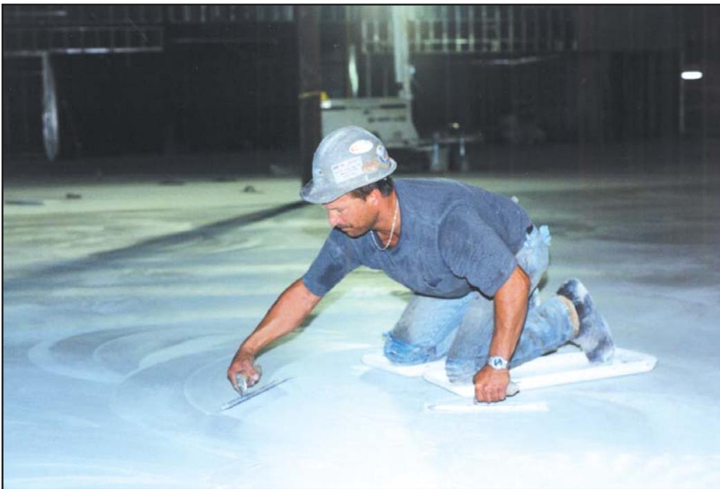
**Figure 8. Hand finishing on the final pass is key to good results. Even with metal tools, trowel burns can be prevented by proper timing. (70175)**
