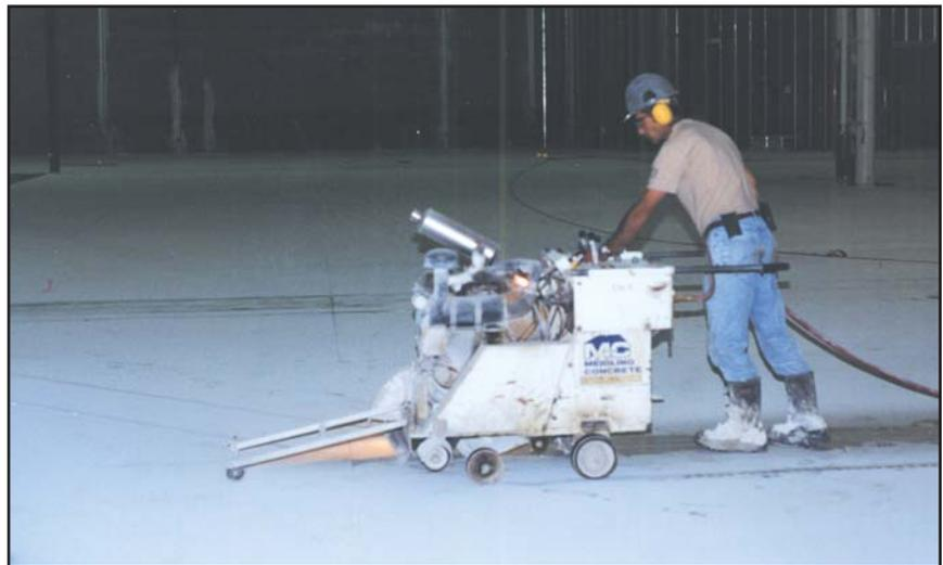
**Figure 5. Because these floors are designed to be seen, no raveling is tolerated during saw cutting of joints. New slabs are generally wet cut the day after placement. (70172)**
