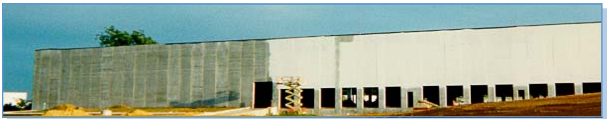
Gray concrete painted white
