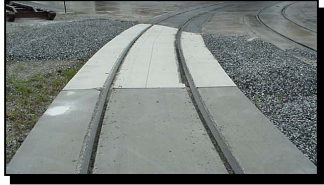
Wet, White Concrete Railroad Crossing
